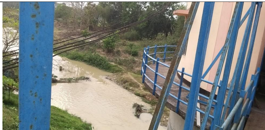
Existing intake on Haora River for Ranirbazar
