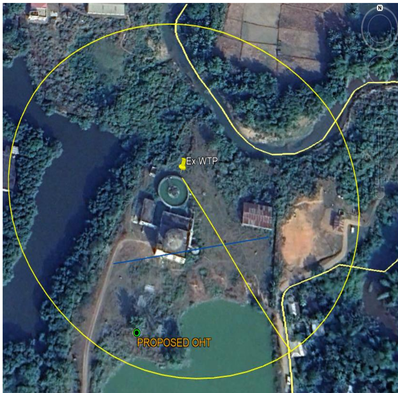
Existing WTP and surrounding 100 m of Khowai
